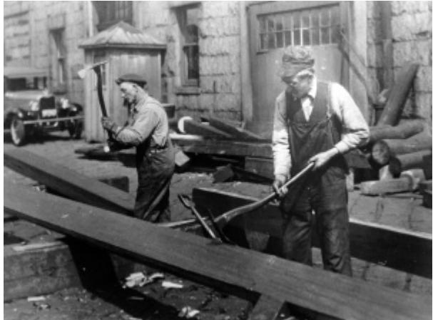
Shipworkers using a Ships Carpenters Adze
